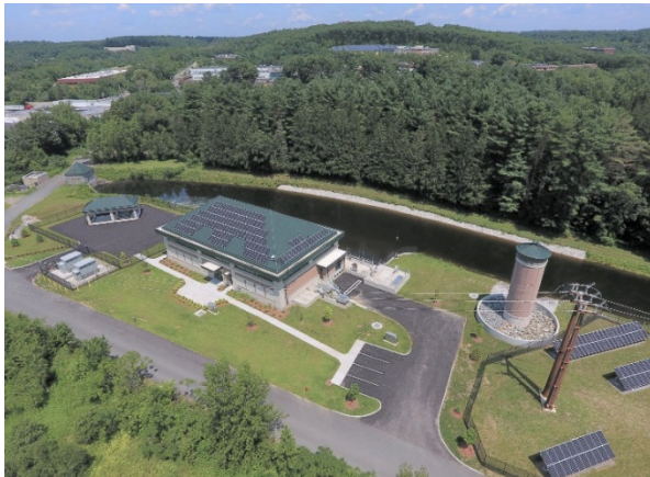
Figure 3 – Wachusett Aqueduct Pump Station Zero Net Energy
