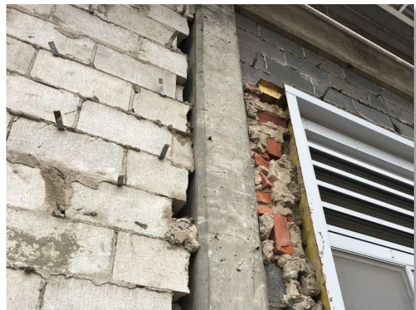
Figure 2 - Headworks Siding Removed
