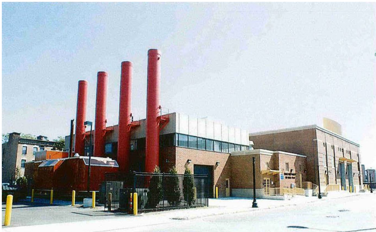
Figure 2 - Exterior View of the Union Park Pump Station/CSO Facility from Malden Street
